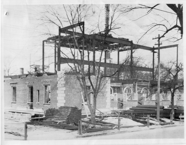
Federal building construction site
