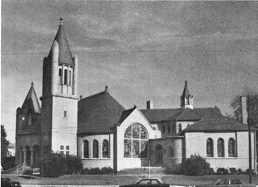
CENTENARY UNITED METHODIST CHURCH, 1992 Photo by Conway.
