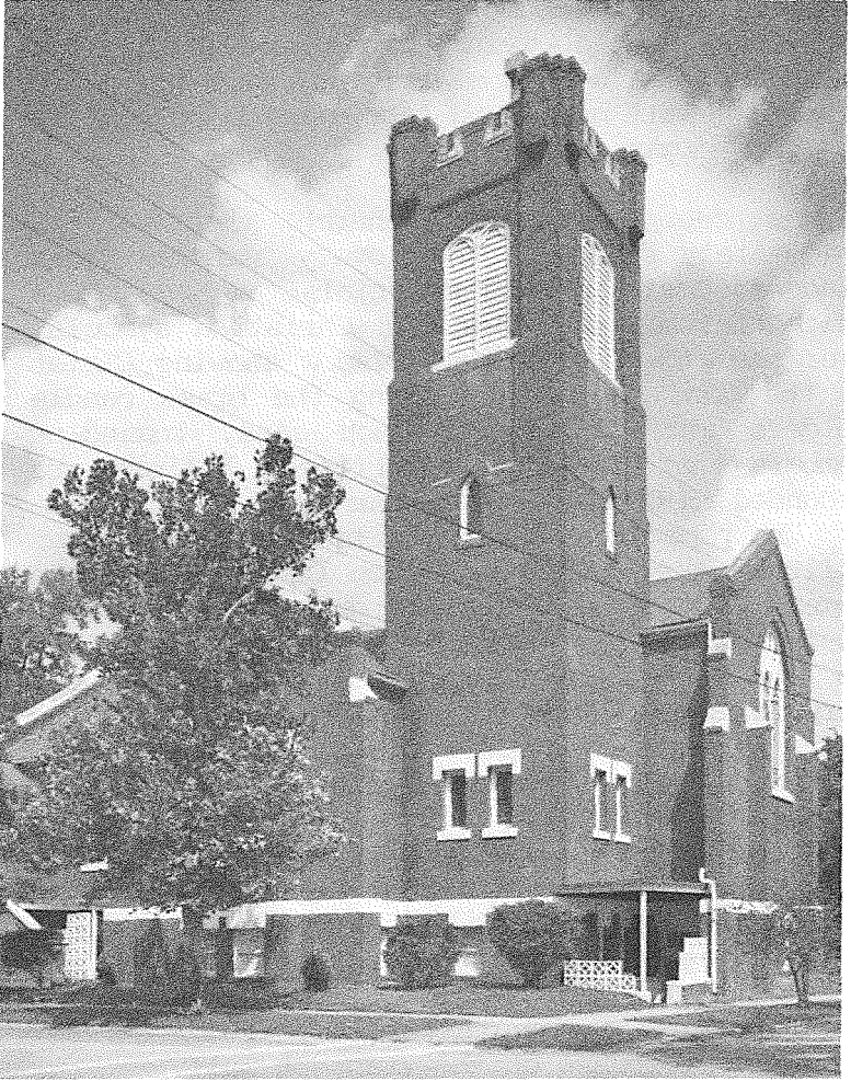
TOWER HIGHLIGHTS ST. CYPRIAN'S CHURCH. Photo by Conway.
