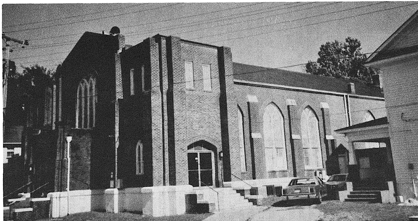
SAINT PETER'S A. M. E. ZION CHURCH STANDS RESTORED AND ENLARGED AFTER THE FIRE OF 1922. Photo by Jim Gunn.
