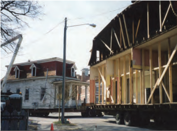
Hugh Lovick House, built in 1898 at 410 Middle Street; relocated to 701 East Front Street in 2003. House had to be cut in half to move it down narrow streets.
