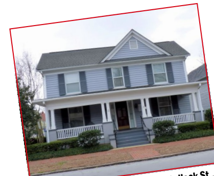
Lawrence /Gaskins House, 601 Pollock St., ca. 1880-1890, owner: Jim Hodges
